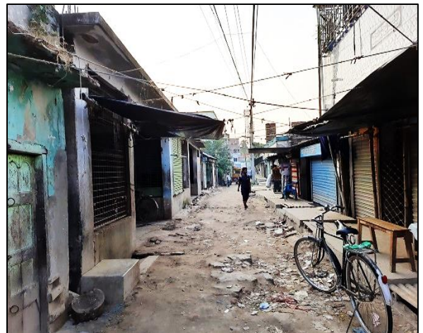
Road -19 and Drain-4
