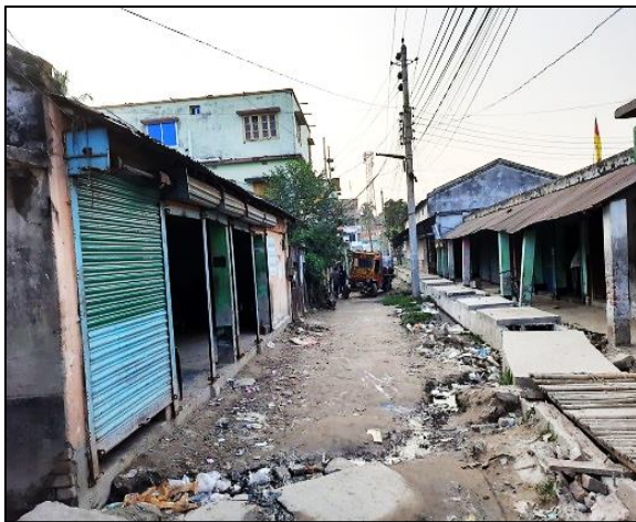
Road -19 and Drain-4
